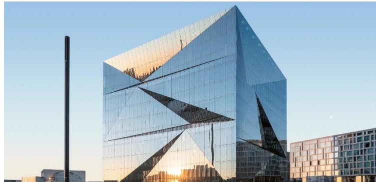
The Cube – Berlin (Germany) Project- and Logistics management, Construction management
