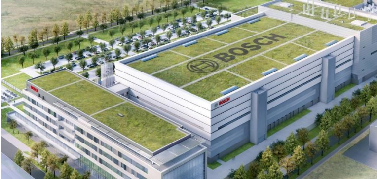
Bosch Chipfabrik – Dresden (Germany) Lean Construction Management
