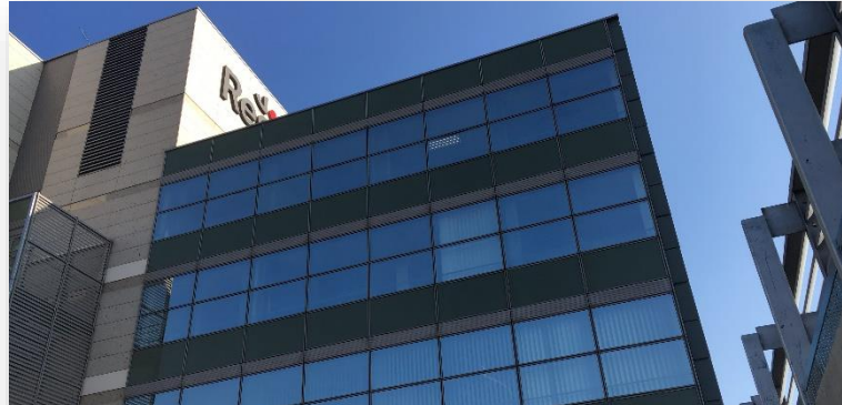
Hoto-Tower – Zagreb (Croatia) Real Estate Consultancy – Technical Due Diligence
